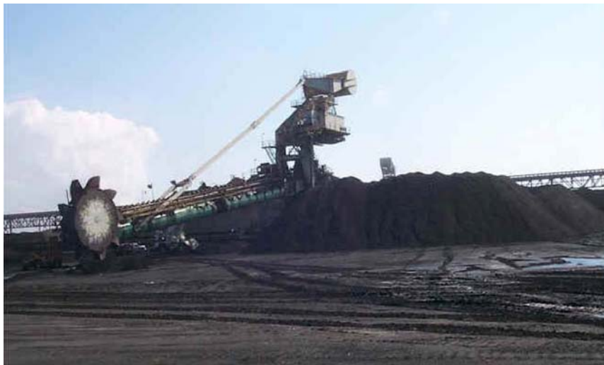
Figure 2. Operations at the McDuffie Island Coal Terminal
